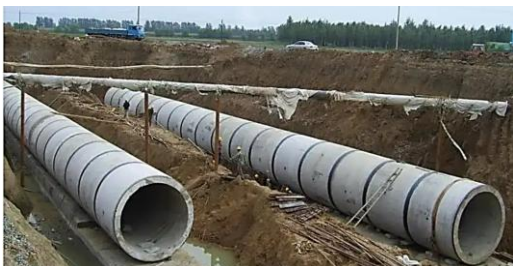
Fig.1. Hydroelectric power station pressure piping
