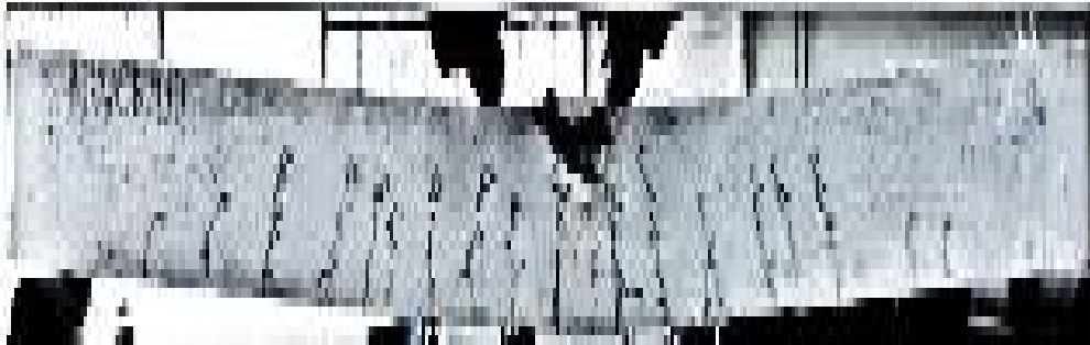
Fig. 5. Typical crack patterns of LFCP 1-3
