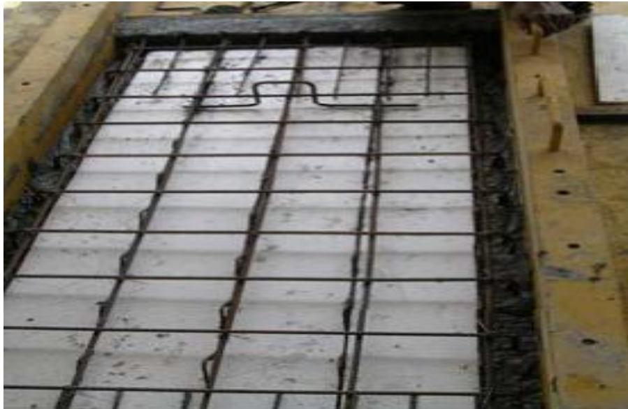
Fig. 2. Reinforcement arrangement of high yield steel 9mm steel and the connector
