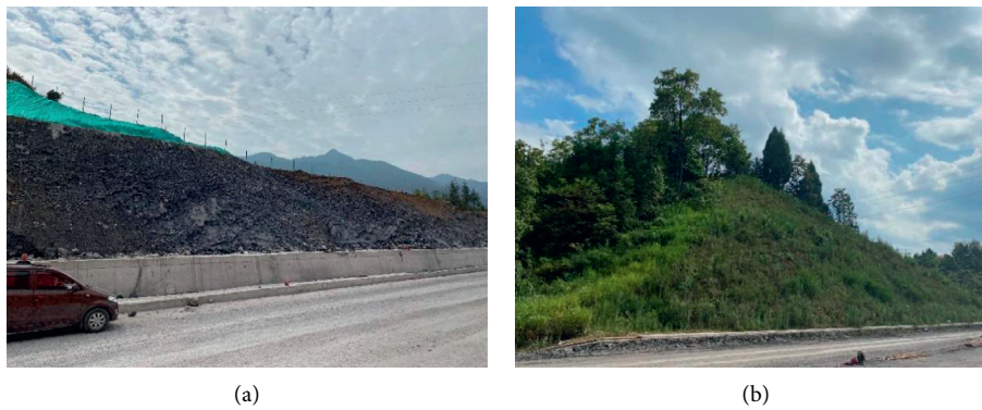
FIGURE 2: Landscape of the studied slope: (a) before slope protection; (b) after planting plants.
