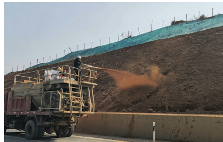
FIGURE 7: External-soil spray seeding.
