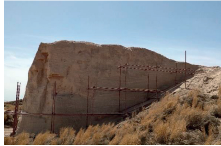
FIGURE 1: The reinforced site wall.
